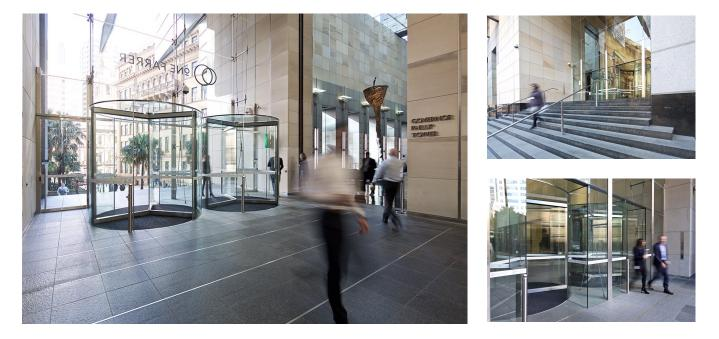
The lobby upgrade to One Farrer Place in Sydney involved replacing the existing 20 year old canopy style revolving doors with new fully frameless record Diamond Series revolving doors as preferred by the architects Johnson Pilton Walker.
