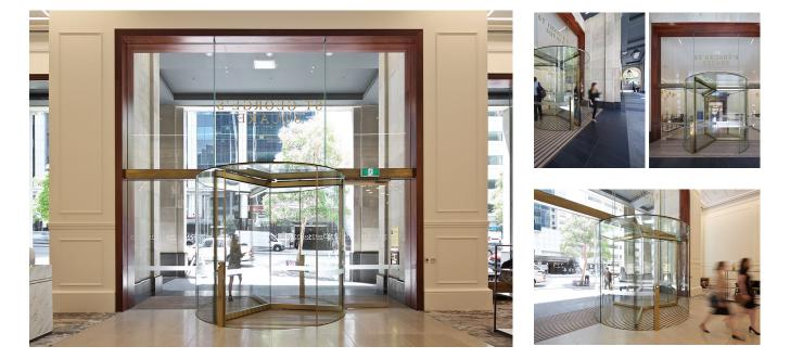
At St George's Square (225 St Georges Terrace) a Grade A commercial building constructed in 1990, a full lobby upgrade was undertaken by FDC Construction with the existing ornate timber revolving doors to both the front and rear entries replaced with sleek all glass Diamond Series revolving doors, specified by Woods Bagot.
